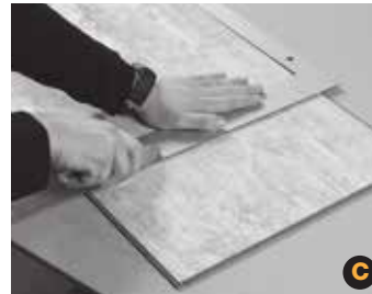
Cut Inspired tiles by scoring and snapping with a utility knife. (image C, D). This method may require sanding the snapped edges.
