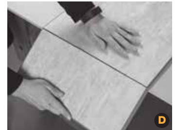
Cut Inspired tiles by scoring and snapping with a utility knife. (image C, D). This method may require sanding the snapped edges.
